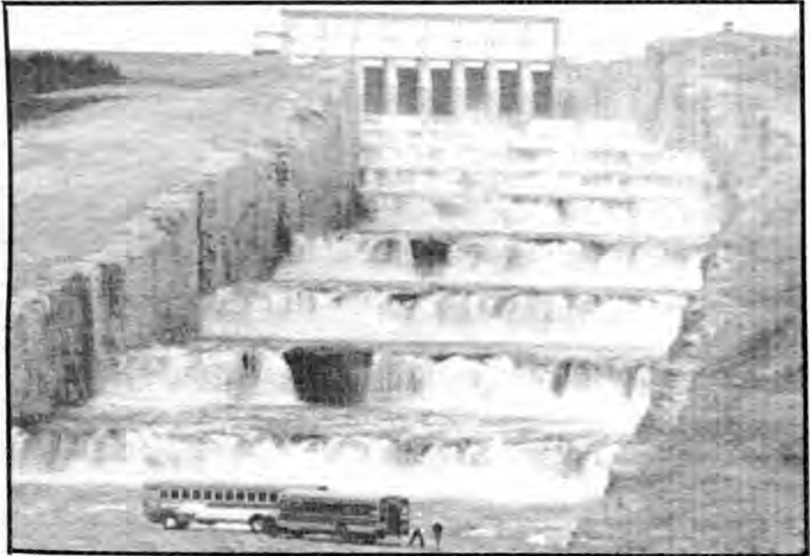
A view of the massive spillway at the LG2 facility on La Grande River in James Bay. This is the water which is
